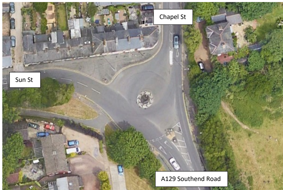
Image 7.66 A129 Southend Rd / A129 Sun St roundabout
