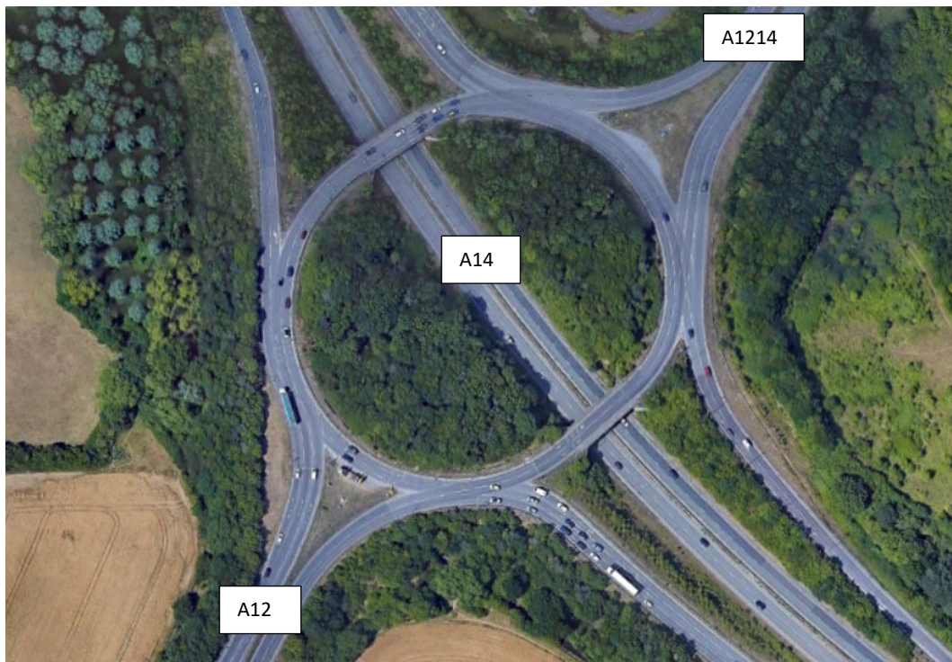
Image 7.6 A14 J55 Copdock Interchange
