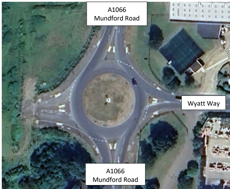
Image 7.33 A1066 Mundford Road / Wyatt Way roundabout
