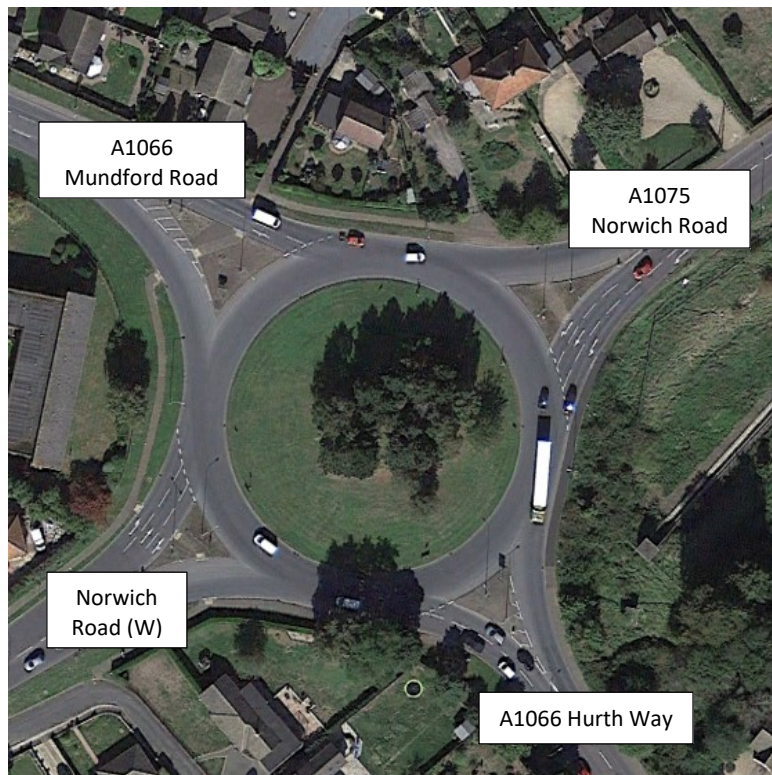
Image 7.34 A1066 Mundford Road / A1075 Norwich Road roundabout
