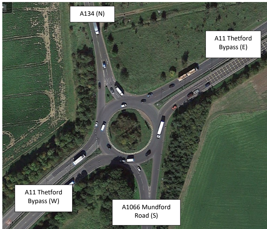
Image 7.2 A11 Thetford Bypass / A1066 Mundford Road roundabout
