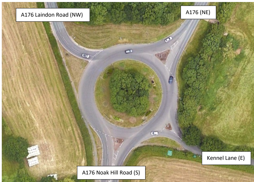
Image 7.65 A176 Noak Hill Rd / A176 Laindon Rd roundabout
